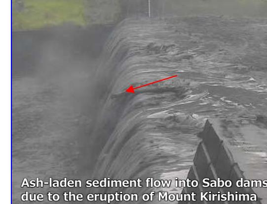
Ash-laden sediment flow into Sabo dams
