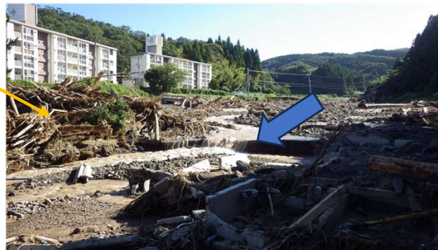
A、B: Sediment and flood damage due to bridge blocked by driftwood
