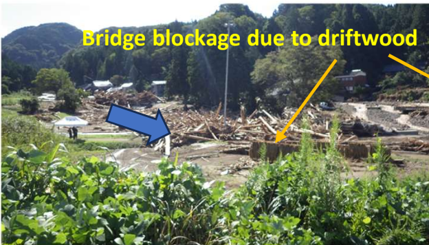
A、B: Sediment and flood damage due to bridge blocked by driftwood
