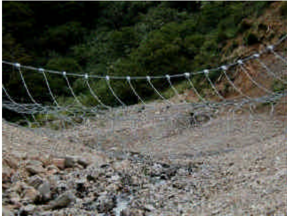
Photo-3 Sabo dam made of Wire Net
