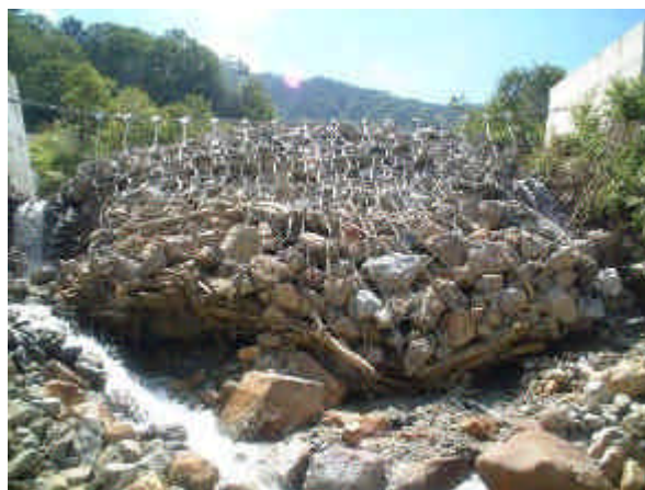
Photo-2 Checking the debris flow in Kamikami-Hori torrent of Mt. Yake dake (Photo supply: Hokuriku Regional construction Bureau, Ministry of Land, Infrastructure and Transport)
