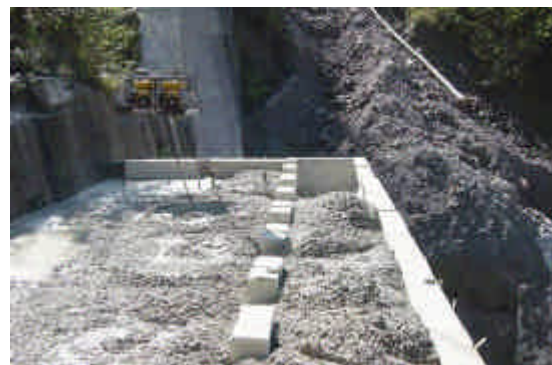
Photo1: Tamping by unmanned vibrator
