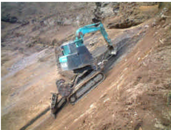
Photo-1 Excavating Work by Rock-climbing Machine
