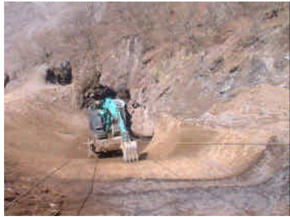
Photo-2 Seeing from the upper part of the slope
