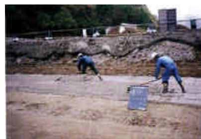
Treatment of construction joint
