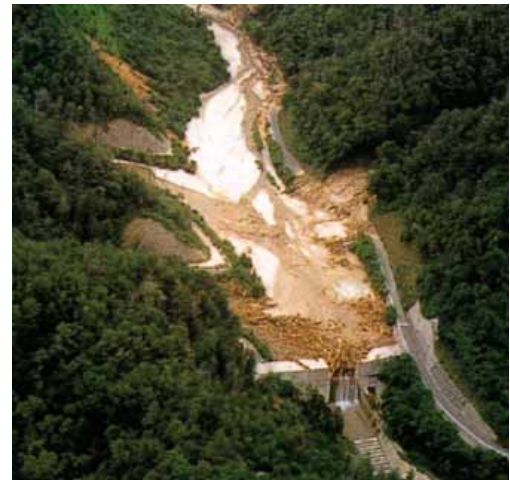
Sabo dam in mid-area of the Aratani River: A debris flow and accompanying driftwood were restrained by this sabo dam in a torrential rainfall disaster that occurred in the coastal area in Hiroshima Prefecture in June, 1999.
