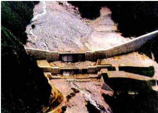
No. 1 sabo dam on the Name River in the Kiso River system: A large-scale debris flow occurred in July, 1989 due to localized torrential rainfall, but this sabo dam prevented it from reaching the downstream.
