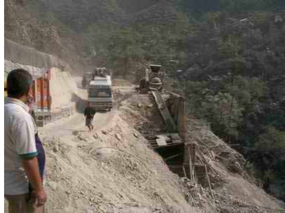
Restoration work is in progress at the Mugling-Narayanghat Road
