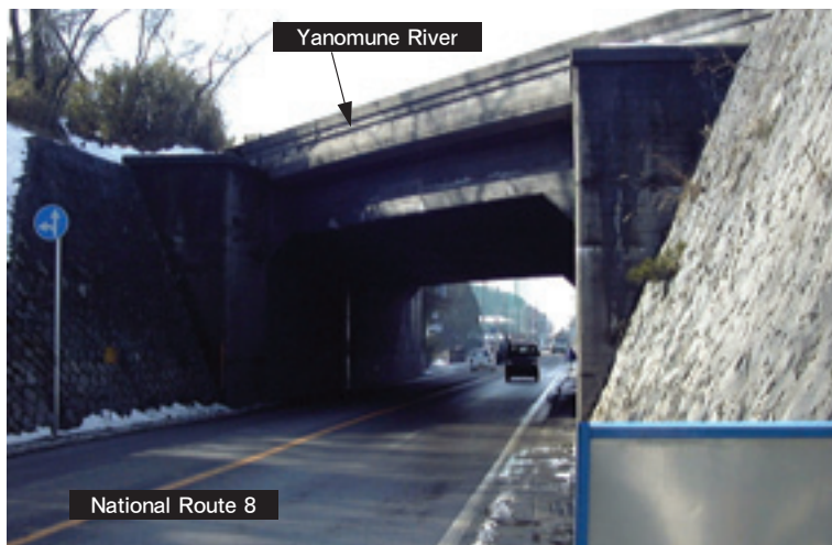
National Route 8 and the Yanomune River running above the route
