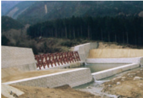
Steel slit sabo dam
