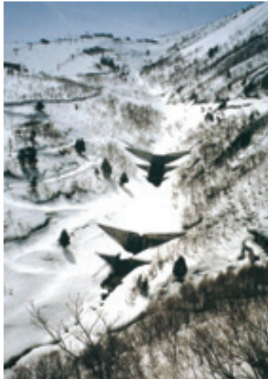
Sabo dam in potential avalanche hazard area (Hakuba Village, Kitazumi County, Nagano Prefecture)
