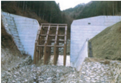
Steel grid sabo dam
