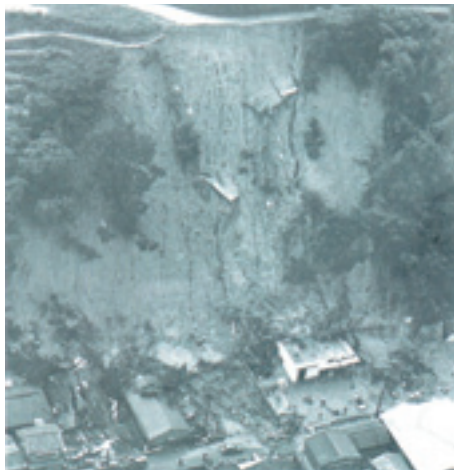
Photo 24 : Slope failure in Kure City (July 1967; Kegoya 8-chome) 21)
