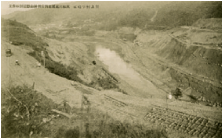
Photo 21: Yamato River new channel excavation (forecasted 16)
