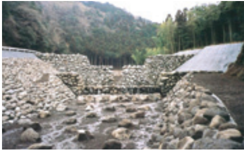
Slit sabo dam
