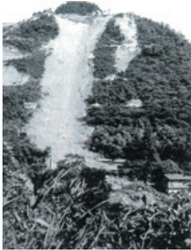
Ichigahara Collapse (Ichigahara, Yamagori, Chuo Ward)
