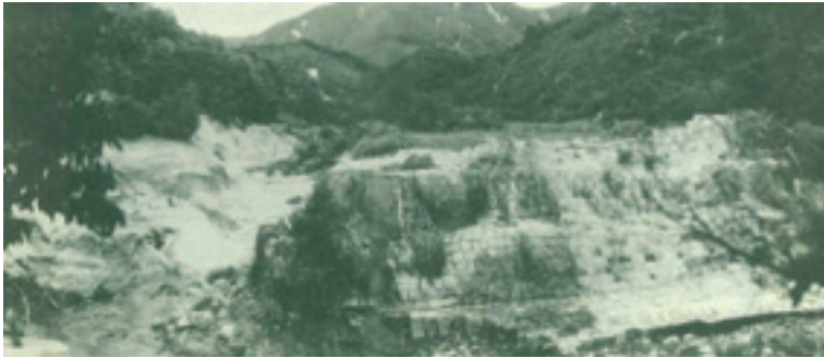
Photo 9 : Hontani Sabo Dam immediately after the Minami Yamashiro Flood Disaster in 1953 7)
