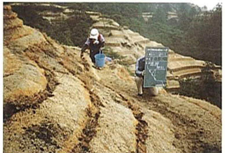
Turf planting and seeding with fertilizer and soil
