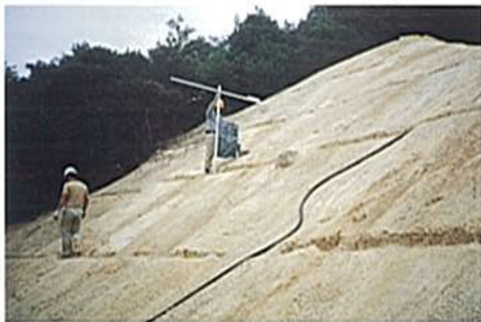
Completion of slope cutting and under making steps
