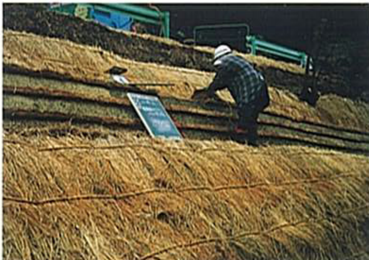
Completion of slope greening and covering
