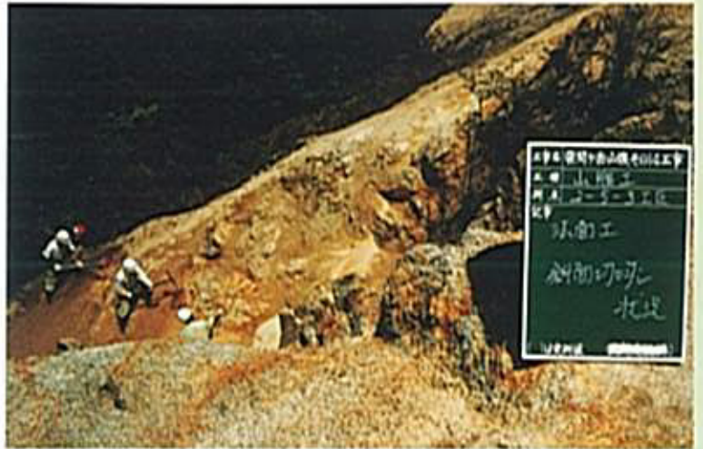
Slope cutting and surface smoothing
