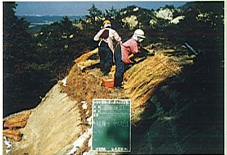
Application of straw mat
