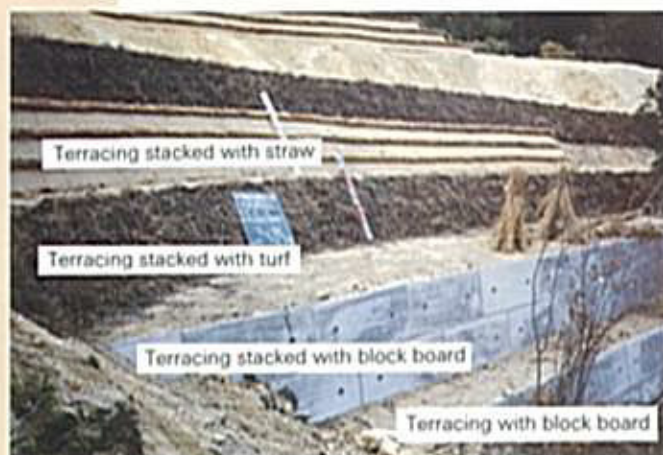
Terracing with block board, and its completion
