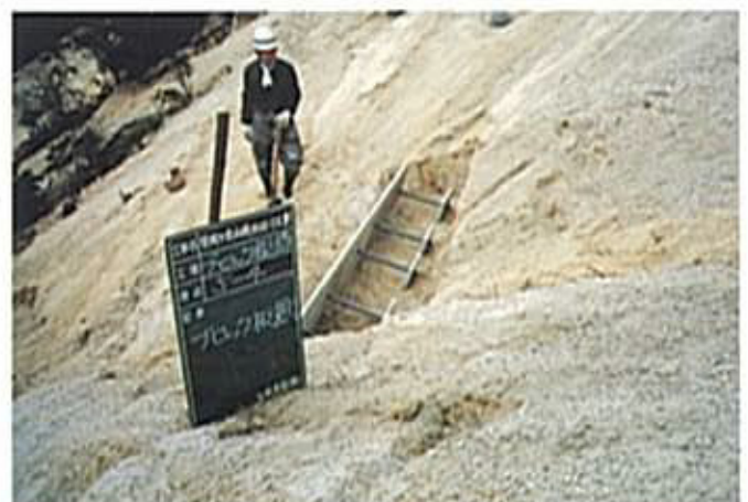
Completion of 1 st block
