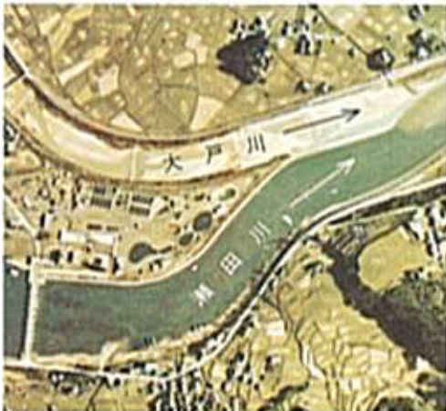
Junction of Daido River and Seta River
