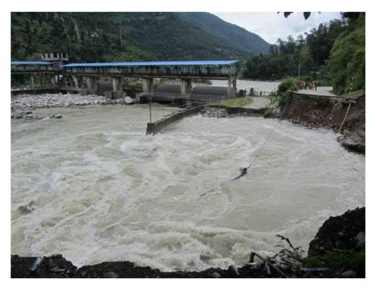
Figure 14: Damaged Sunkosi Hydropower Headwork and Araniko Highway after breach of the Landslide Dam
