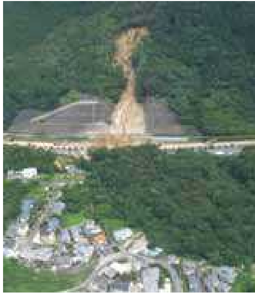
Slope failure hit a village. ( Otogane, Onojo City)
