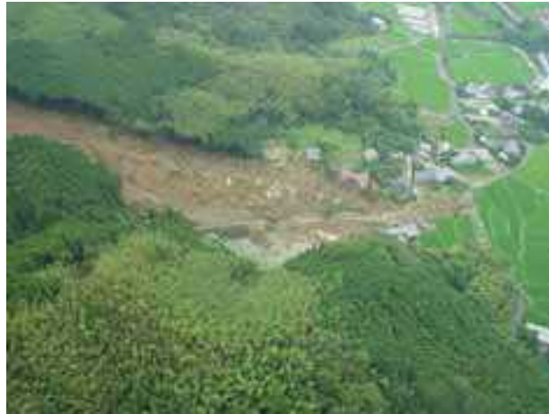
Hillside collapse hit a village. ( Benjou, Fukuchi Town)
