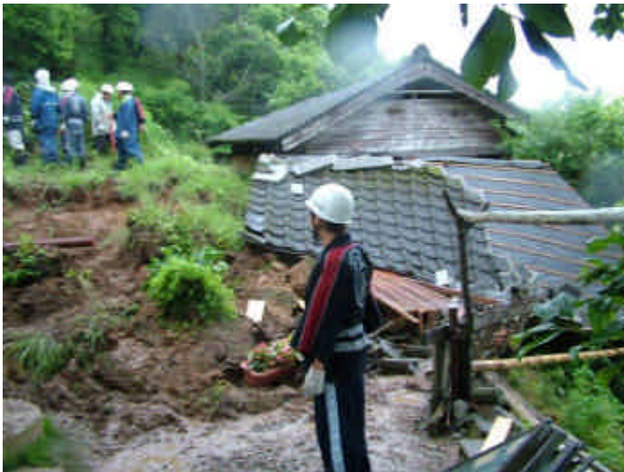
Steep slope failure occurred, and the residence was destroyed by this disaster (1 dead).
