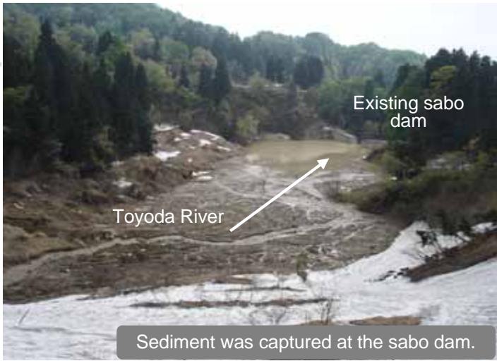
[May 10, 2005: landslide] Place: Urada area, Tokamachi City, Niigata Prefecture Damage: A landslide occurred in the area of 70 m wide and 300 m long. The Toyoda River (sabo river) was clogged with sediment.
