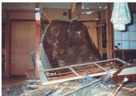
Photo 1. Damage due to the boulder plunged into the house
