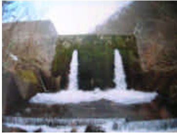
3rd Sabo Dam
