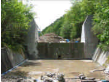
Crest of the dam
