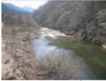
Sedimentation in the 3 rd dam reservoir
