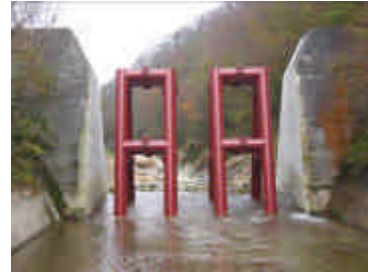
Completion of the work
