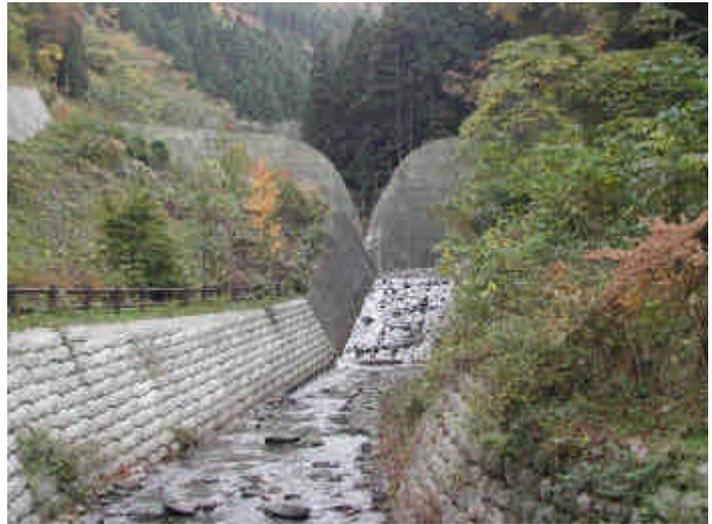
The slit sabo dam and protection wall
