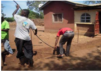
Works to bury the cable in the ground (Kenya, 2013)
