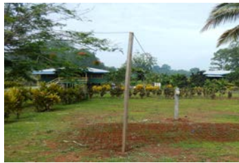
Cable hanging high above the ground (Solomon Is., 2016)
