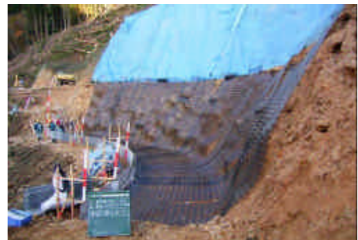
Situation of the footing net
