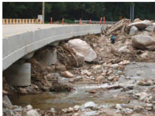
Photo-3 Bridge closed with rocks and driftwoods; Bridge beams displaced by 30cm (Buk-Hangye)
