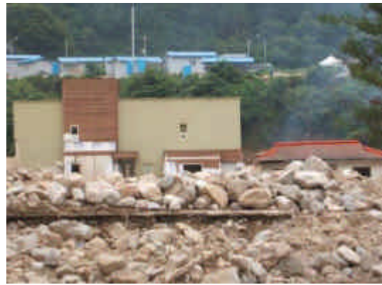
Photo-5 Damage to houses at Buk-Hangye
