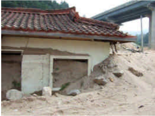
Photo-1 Damage to Soksa 1-ri
