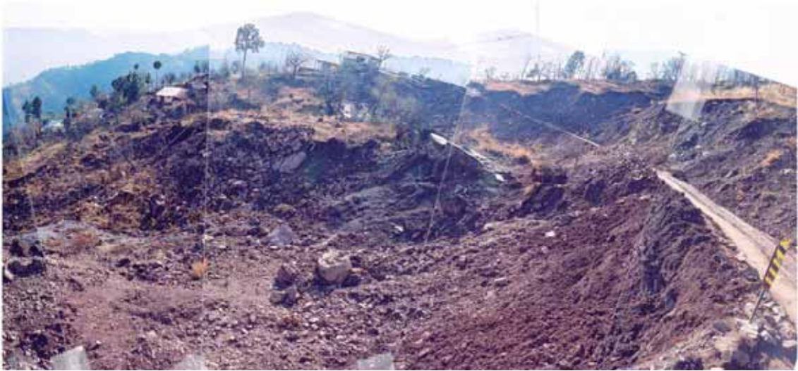
Photo-1 Collapsed roads due to landslide
