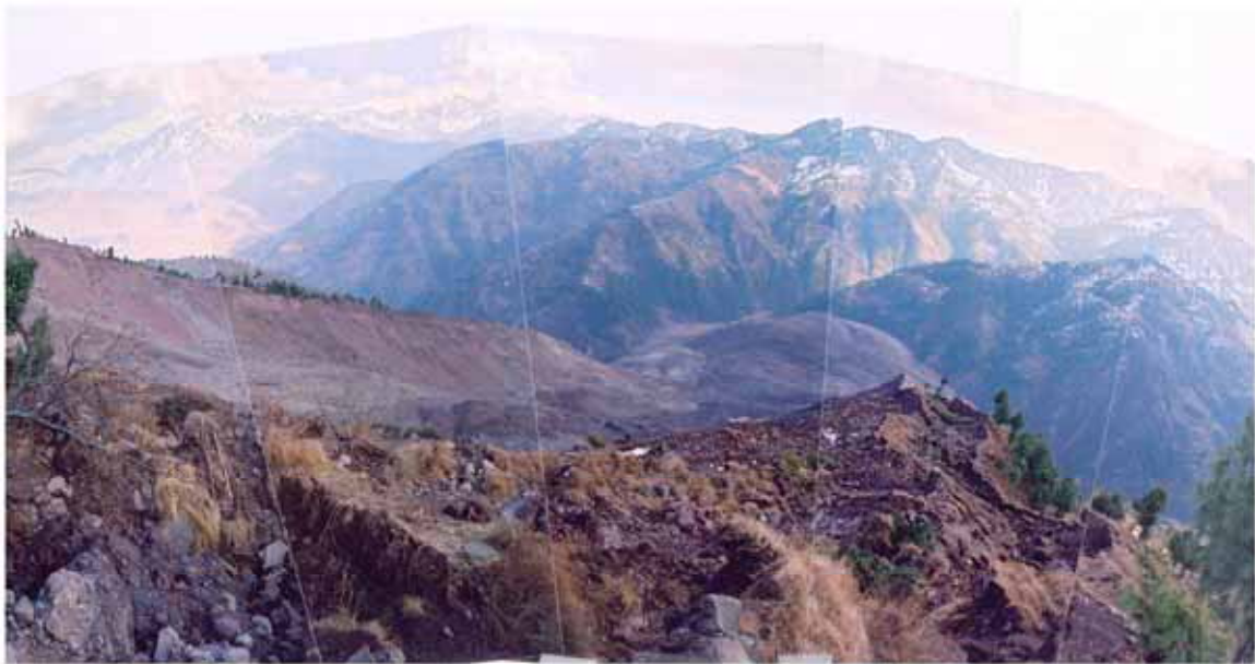
Photo-2 Hathian landslide (Seeing the landslide area from the side cliff at the upper side)
