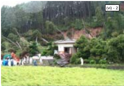
<(vi) Kiriyoze Area, Mimata Town, Kitamorokata Gun (Killed: 2) Landslide>
