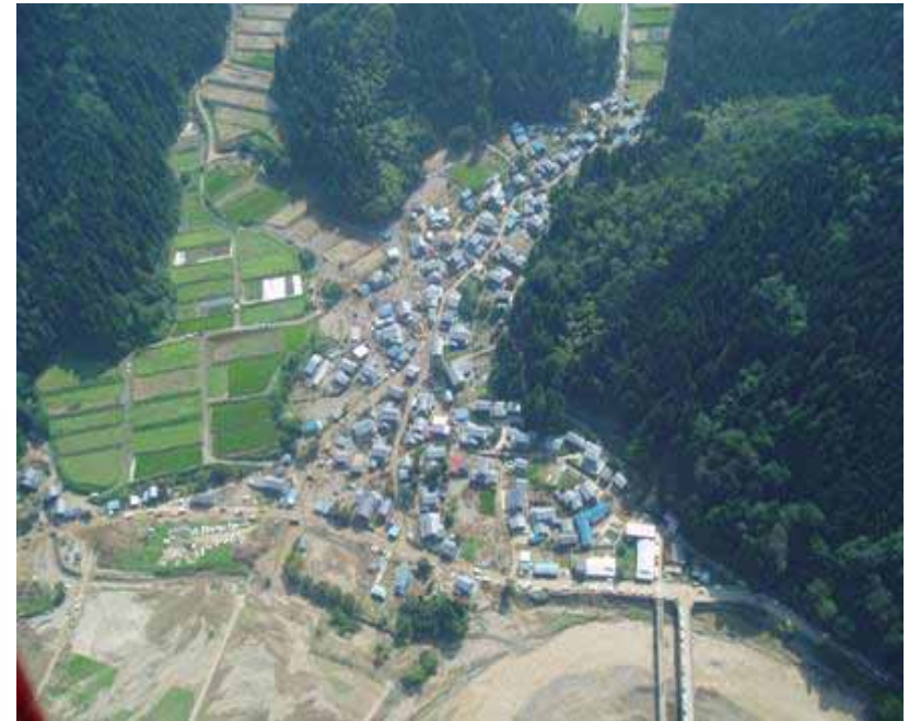
Kuratsukuri, Miyama Town, Asuwa Gun, Fukui Prefecture (total collapse: 12)
