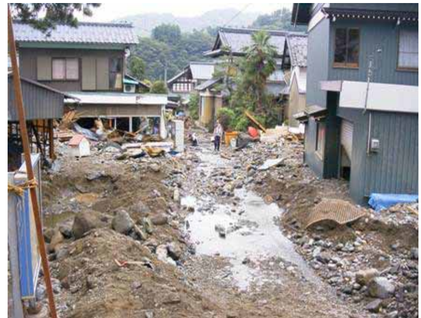
Kuratsukuri, Miyama Town, Asuwa Gun, Fukui Prefecture (total collapse: 12)
